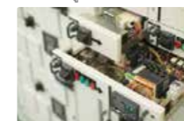
Direct connection to the vertical busbar (IPxxD)
