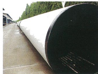
Cooling water pipe
