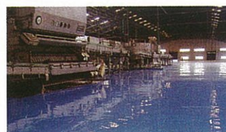
Epoxy floor coating
