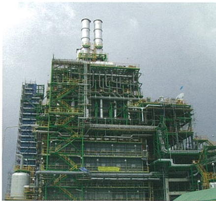
PTT PETROCHEMICAL PLANT
