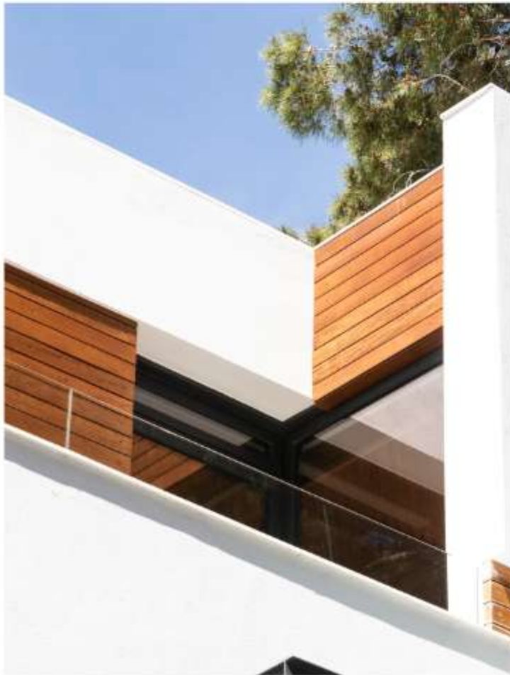
Reference Idea Dura+ Wood Cladding Weather Groove Natural SYP 12x95x2440-4880 mm SYP 15x132x2440-4880 mm
