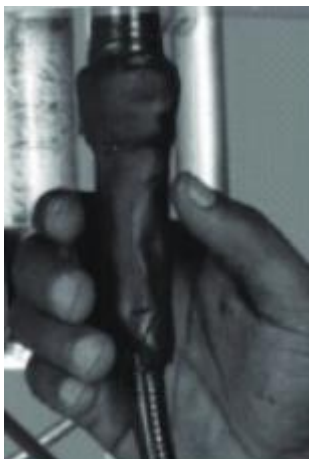
Figure 2-3 Wrapping Waterproof Clay
