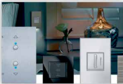
Electrical installation control
