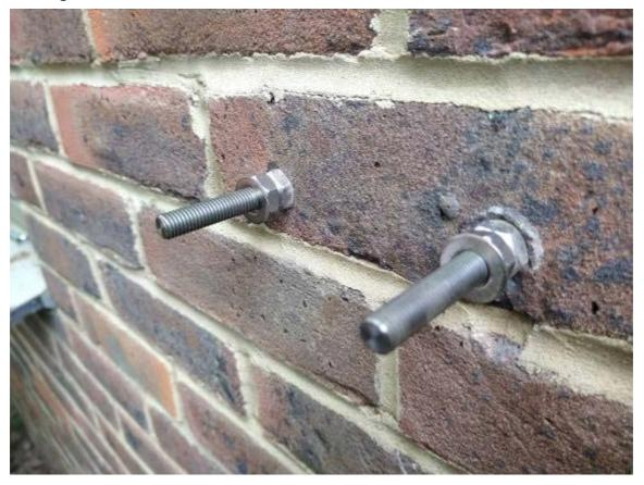
Position the base plate over the anchors.
