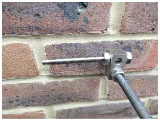
Cut the wire 15mm past the end of the wire tension stud.
