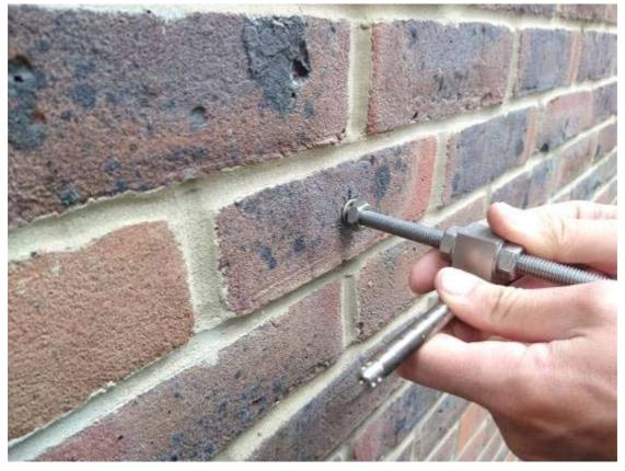
Adjust the anchor to the desired position and orientation and then lock in position by tightening the two securing nuts.
