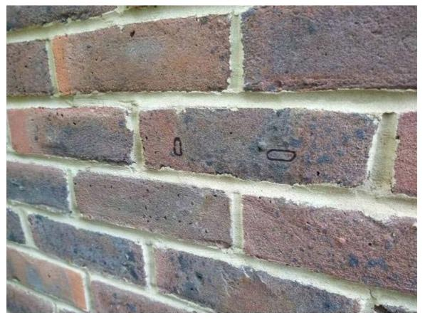
Drill to the depth of the anchors using the 16mm diameter masonry drill in the centre of the marks.
