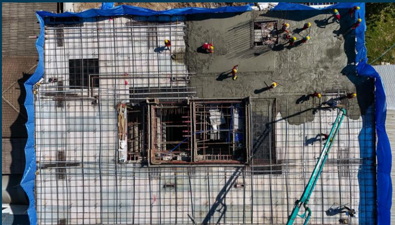
Survey the building construction
