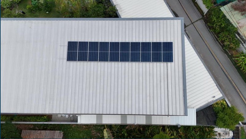
Survey the installation of solar cells
