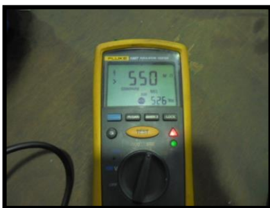
Fig 46. Insulation V1-G Test
