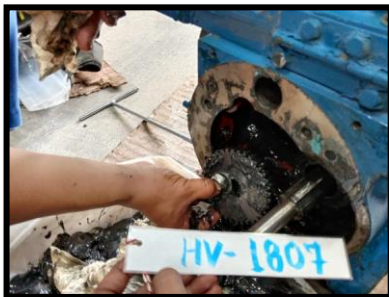
Fig 13. Inspect Gear Shaft Motor
