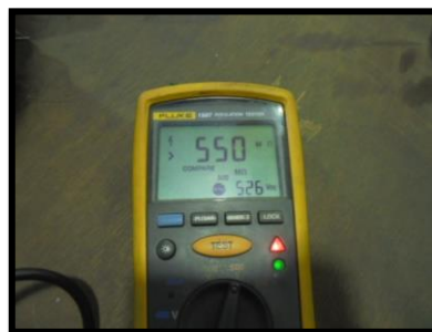
Fig 47. Insulation W1-G Test
