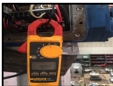
Fig 4. Current of Phase 3 (Before)
