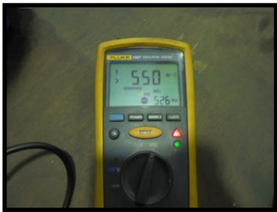
Fig 46. Insulation V1-G Test
