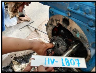
Fig 13. Inspect Gear Shaft Motor
