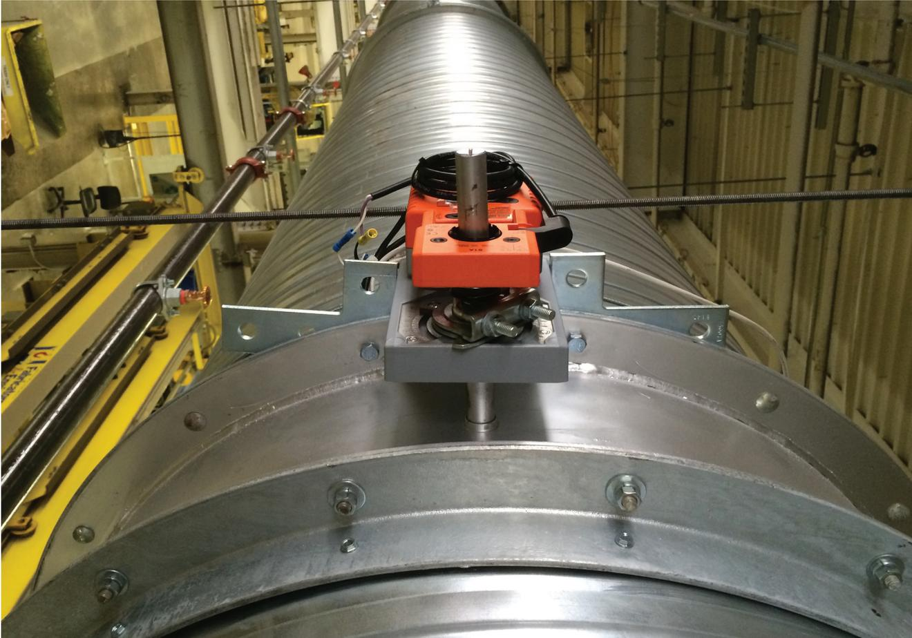
Belimo damper actuators are designed for use in a wide variety of HVAC applications for ensuring performance, reliability, and lower power consumption. Our comprehensive torque range (9 to 1,400 in-lbs) is suited for damper sizes as small as 4-inch round allowing the ability to mount on standard damper shafts or directly on jackshafts. Actuators are used for control dampers, air handlers, economizer units, VAV terminal units, fan coil units, fan shutters, and unit ventilators.
