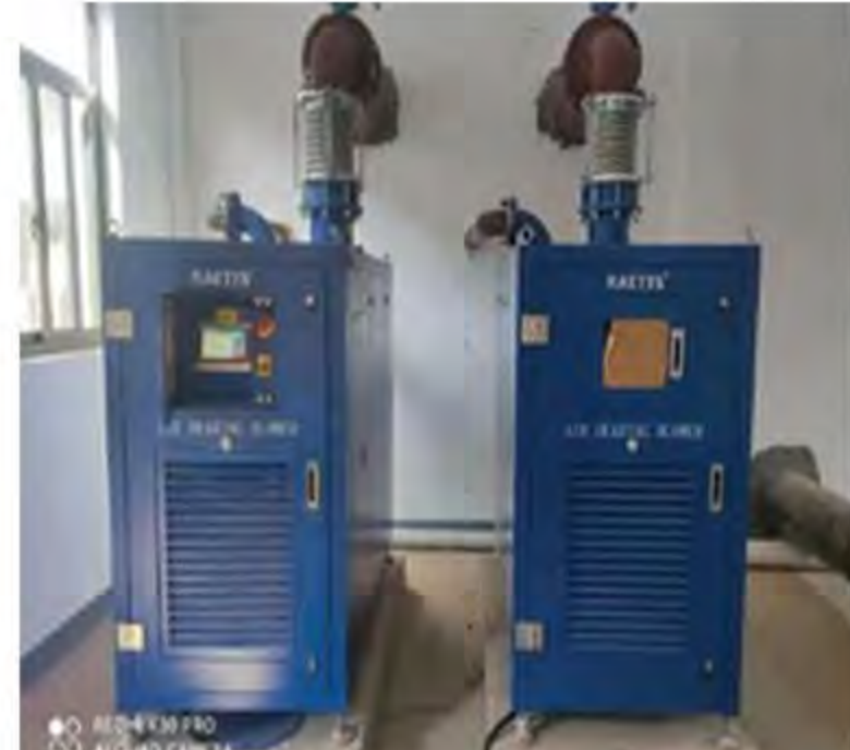
Sewage treatment factory in Changxing Hongqiao
