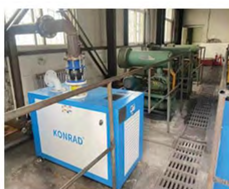
coal industry Sewage treatment factory
