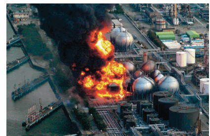
An explosion incident in hazardous area
