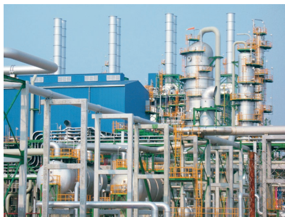
Potentially explosive atmosphere within a process area
