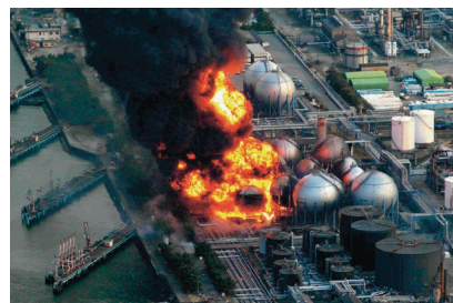
An explosion incident in hazardous area
